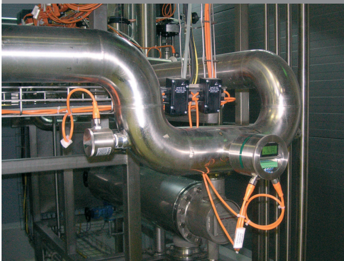
Phase separation in CIP-equipment with ILM-2
